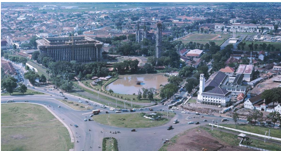
Masjid Istiqlal under construction in 1963 (Collection Nationaal Museum van Wereldculturen)
